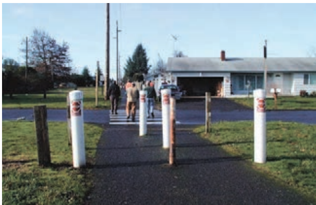
Bollards are overused and can cause injury
