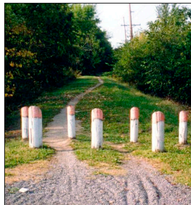
Too many bollards inhibit path access.
