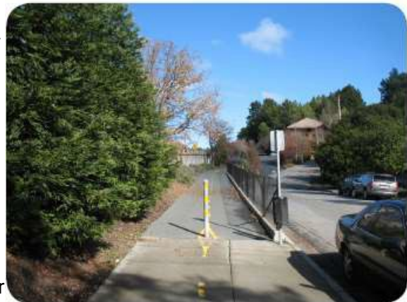
Bollards and pavement change prevent motor vehicles from using the trail.
