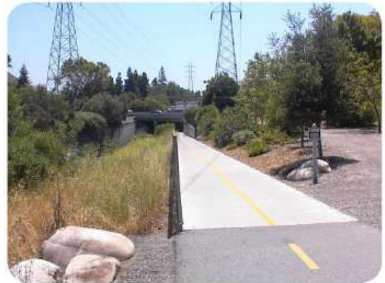
Centerline striping encourages trail users to provide space for other users to pass.
