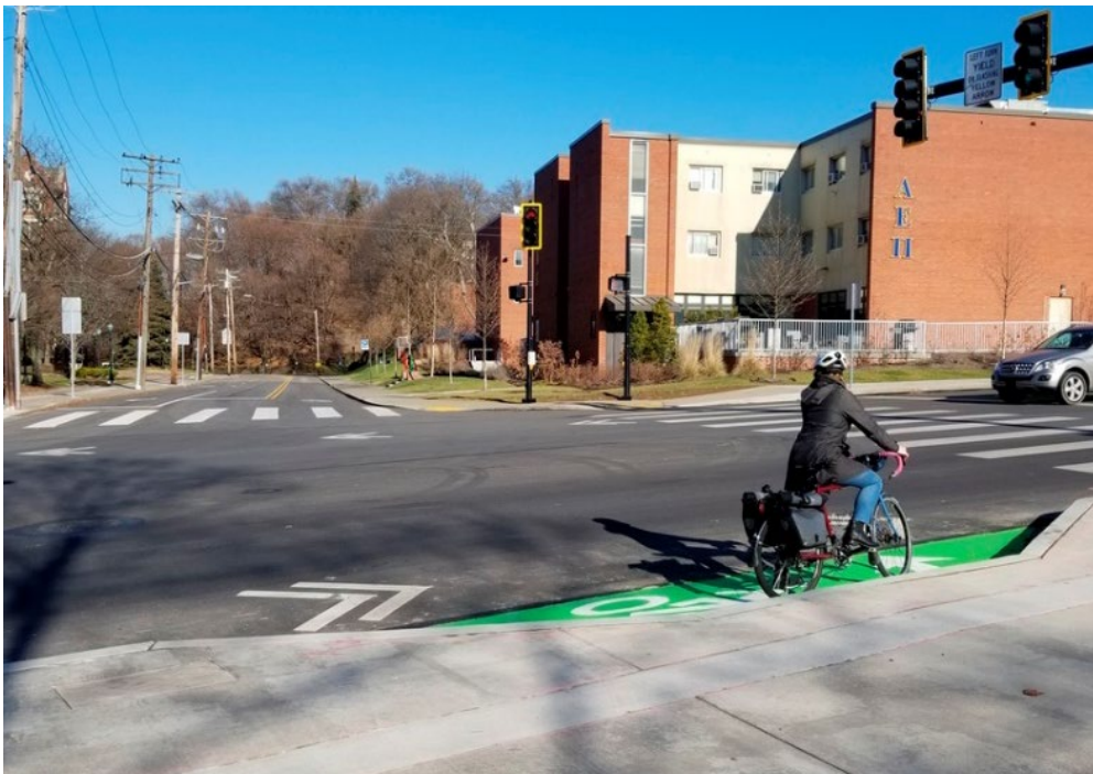
Figure 13: Example of a Two-Stage Bicycle Turn Box
