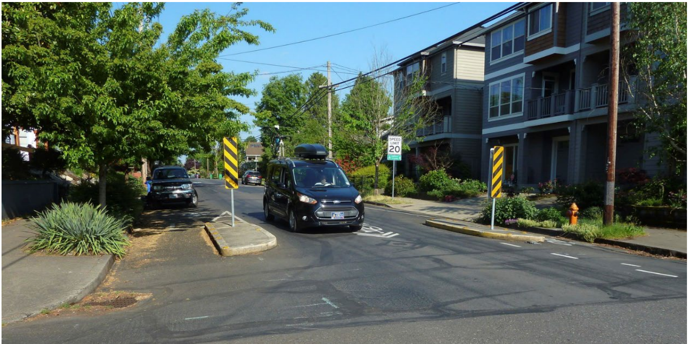
Figure 17: Example of One Lane Pinch Point
