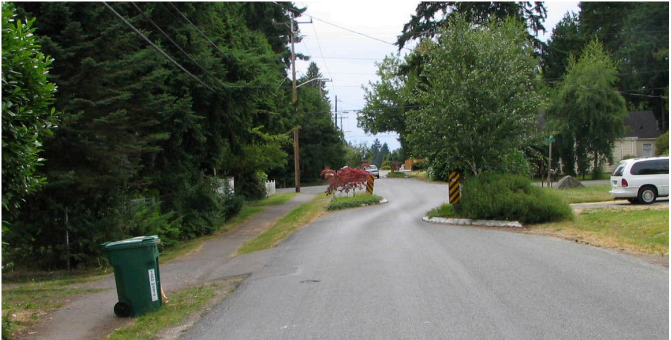
Figure 18: Example of Chicane Use as Traffic Calming Treatment
