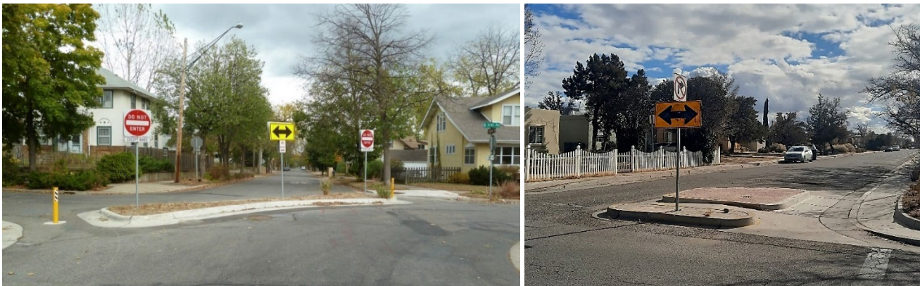
Figure 23: Example of Diagonal Diverter and Partial Street Closure with Bicycle Cut Through along Local Street
