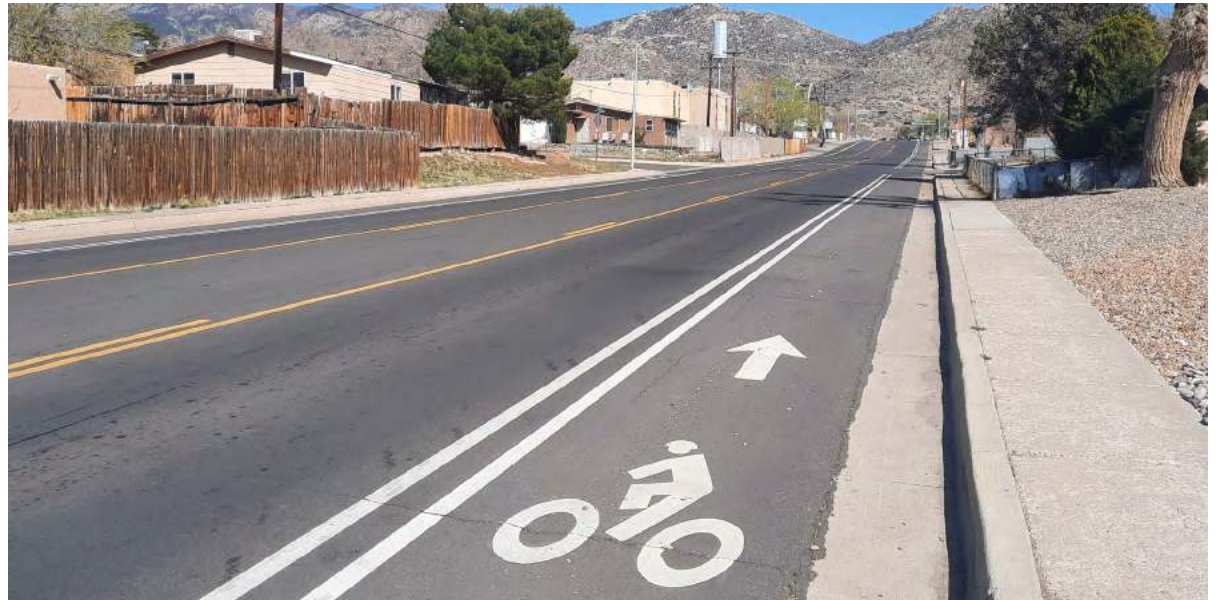
The travel lanes on this section of Copper Avenue east of Chelwood Park Boulevard were recently narrowed to create space for a striped buffer.
